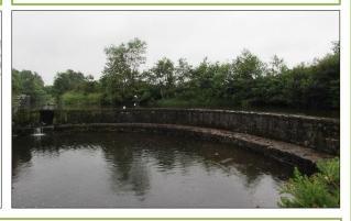
**Historical 25" map** drawing of a weir on the Nore (photograph on the right) known as "The Basin". This weir was constructed in the late 1800s. Like many fish passes built at that time, the pass shown in this map is specifically designed for salmon and may not work for other native species (e.g eel, river lamprey, sea lamprey and cyprinids).
